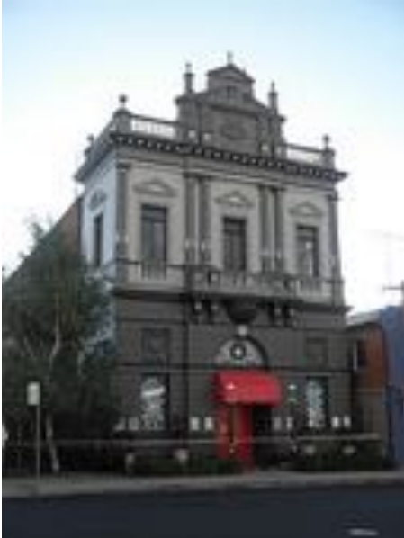
Italianate style stuccoed and decorated surfaces on the façade of the former Masonic Hall, built 1889.
