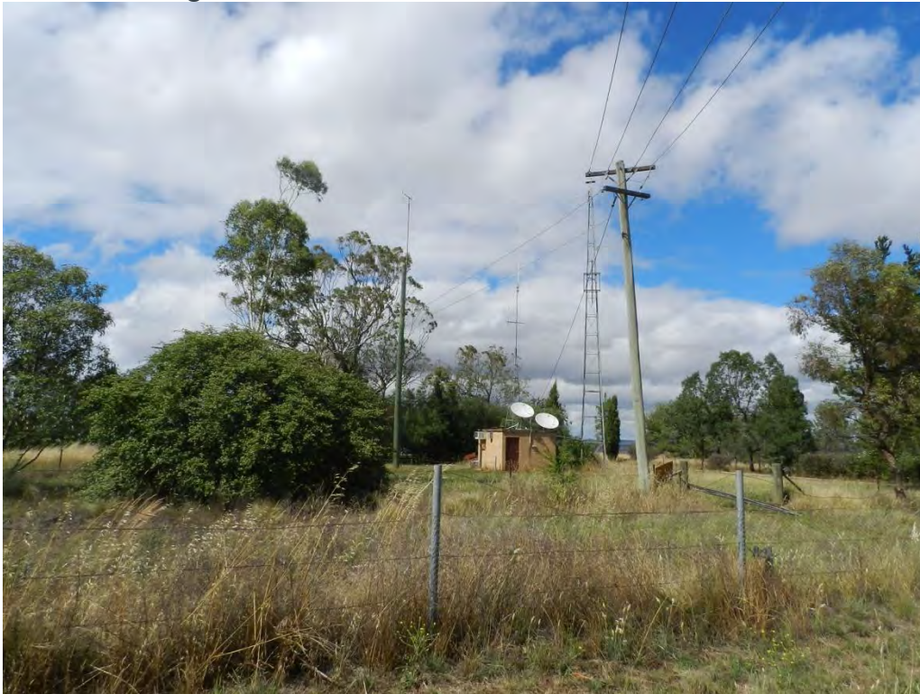
Photo 4: Existing infrastructure to be removed
