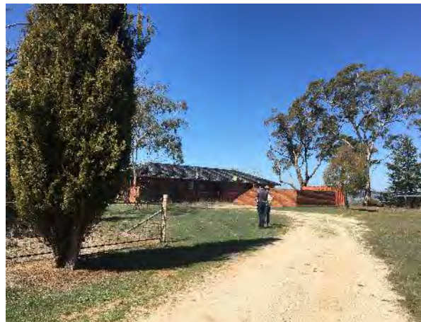
Plate 8 Unoccupied residential house
