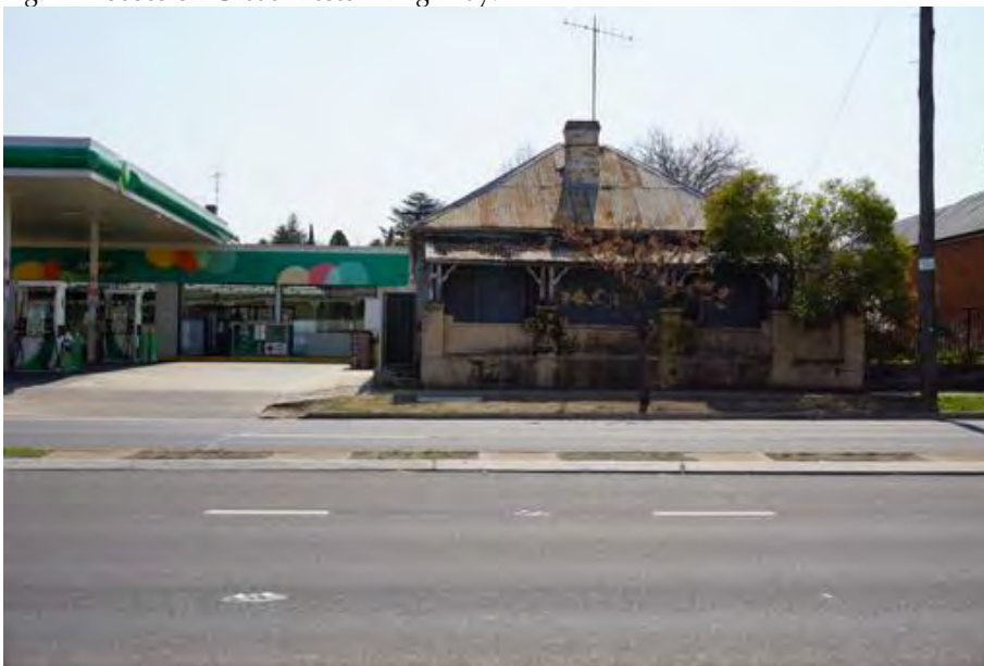
Fig.12 House on Great Western Highway.
