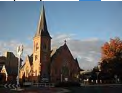
St Stephen's Church, built 1872.
