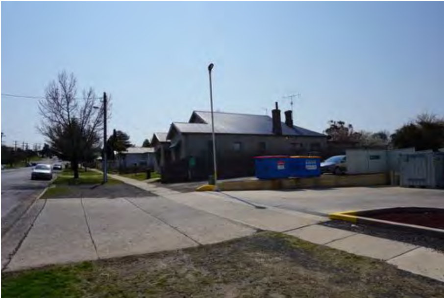
Fig.19 View to No. 261 from outside the service station on the corner of Lambert Street and The Great Western Highway.
