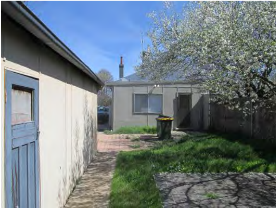
Fig. 29 Garage and rear door of the existing building
