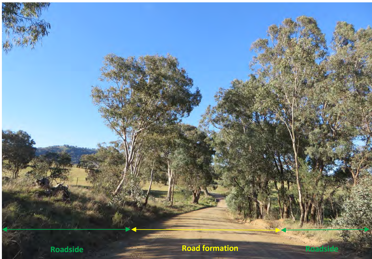
Figure 3-1 Areas of the road formation and roadside within the road reserve
