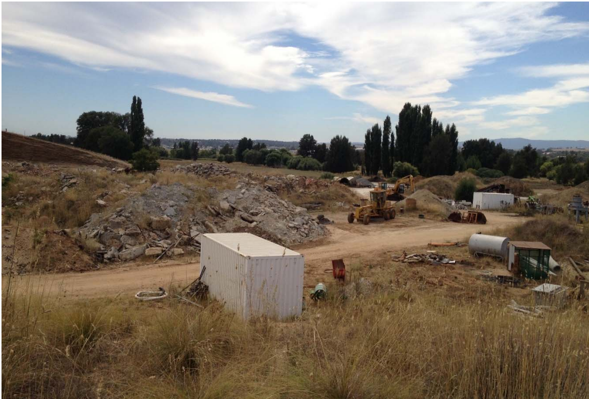
Plate 2 – Existing quarry looking to the north east
