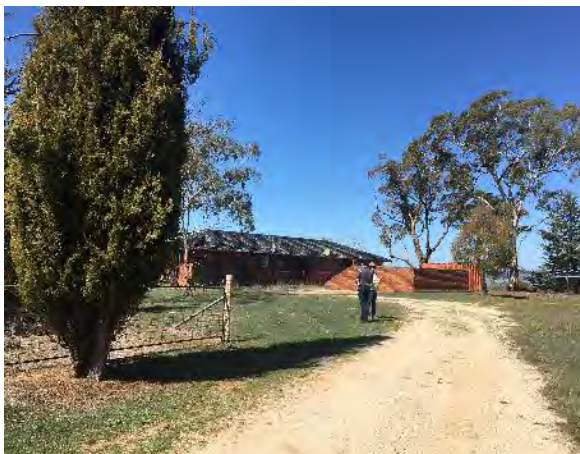
Plate 8 Unoccupied residential house
