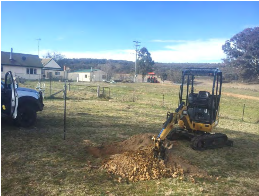
Image 1: Subsoil investigation at the proposed development site
