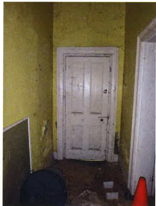
Fig. 9 Rear door in hallway.
