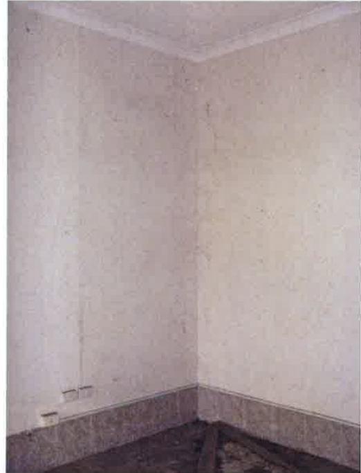
Fig. 27 North section of building.
