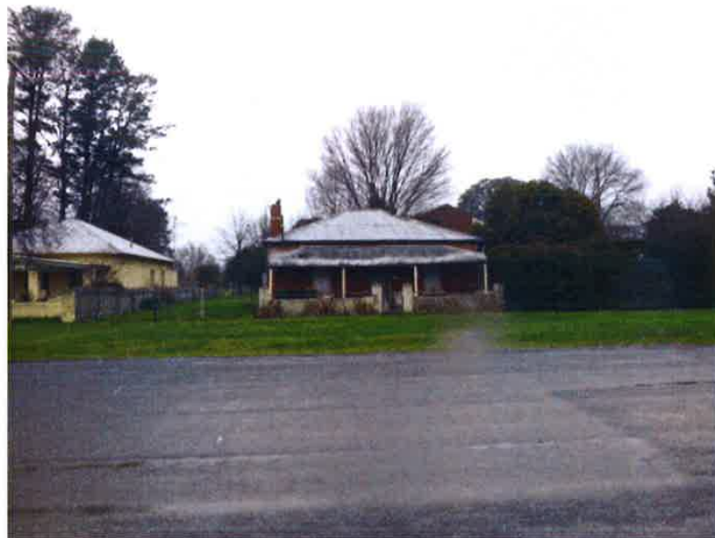
Fig. 59 Houses Baillie Street
