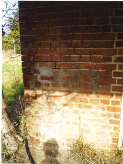
Photo No. 11: Rising damp visible, mortar failure.
