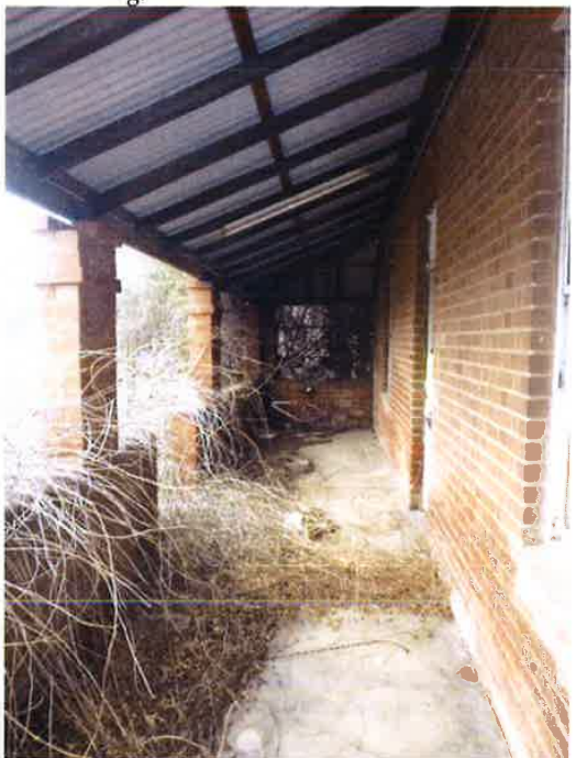
Fig. 19 Veranda The original veranda has been replaced with brick posts and balustrade. The veranda is reroofed and the floor resurfaced Fig. 20 Veranda
