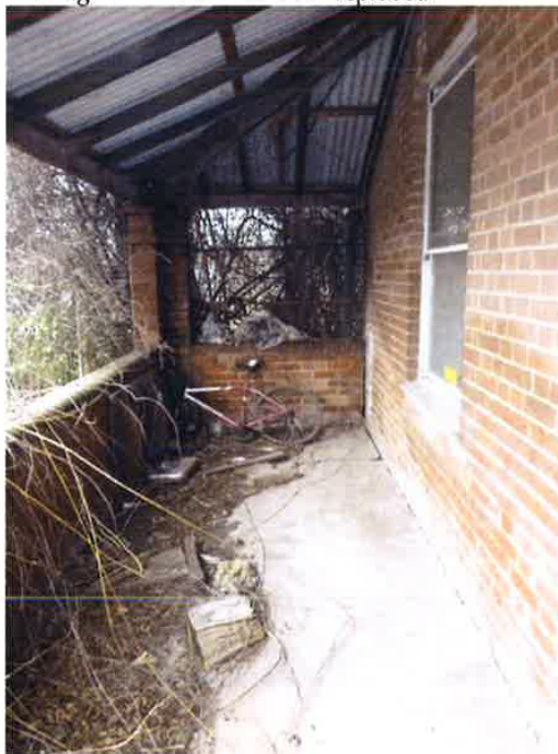
Fig. 19 Veranda The original veranda has been replaced with brick posts and balustrade. The veranda is reroofed and the floor resurfaced Fig. 20 Veranda
