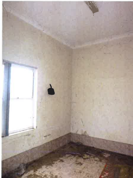
Fig. 28 North section of building.
