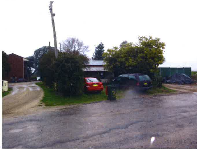
Fig. 60 Houses Baillie Street
