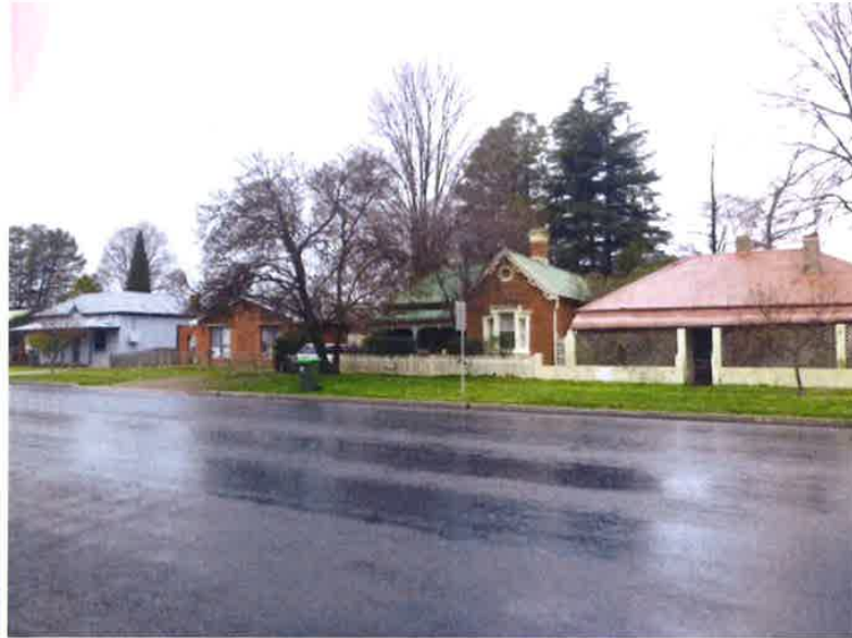
Fig. 50 Three Victorian houses with a contemporary infill on Havannah Street between Baillie Street and the Great Western Highway.
