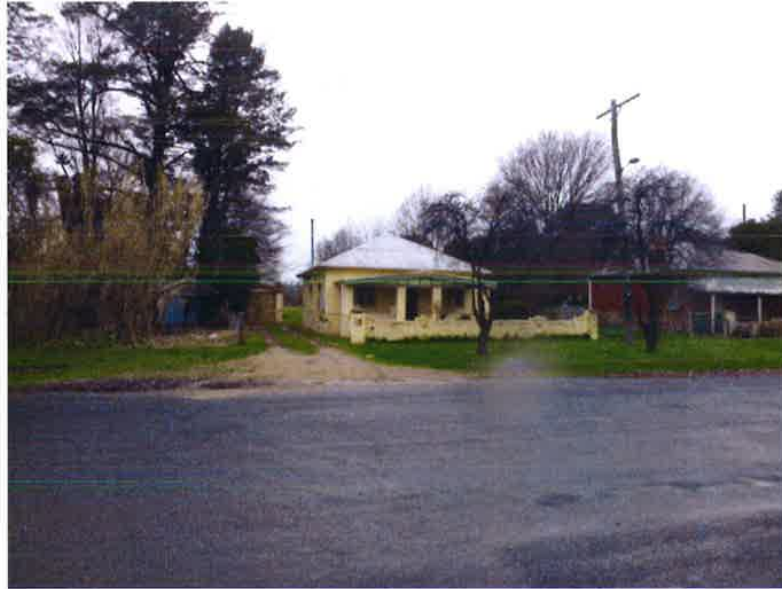
Fig. 58 Houses Baillie Street
