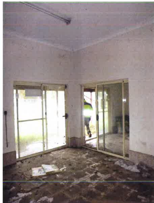
Fig. 25 Floor has been tiled.
