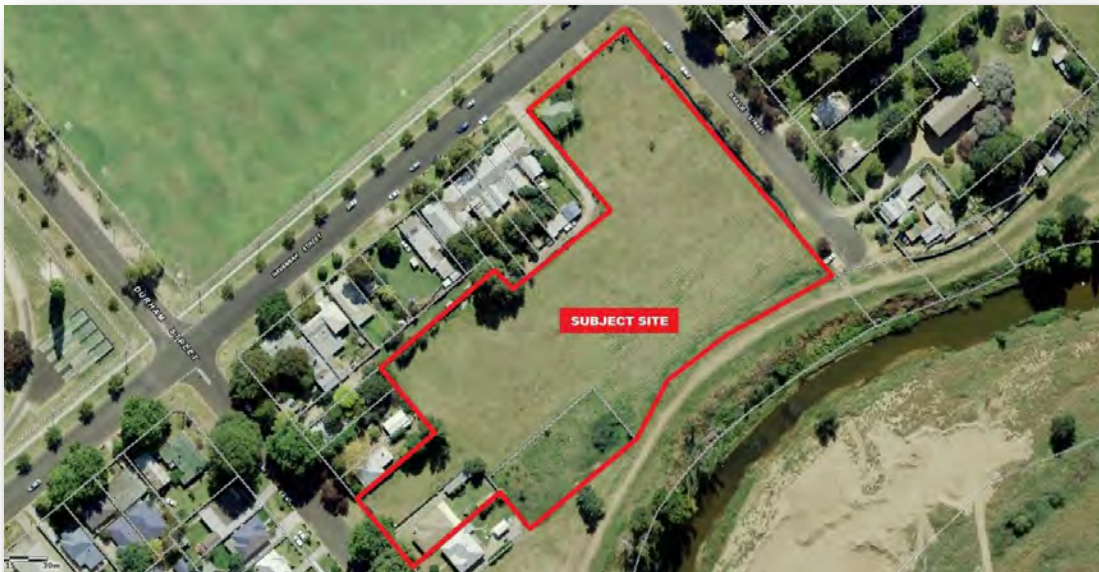
Figure 3 – Aerial Photograph of Site Source: (NSW Government Spatial Services, 2019)
