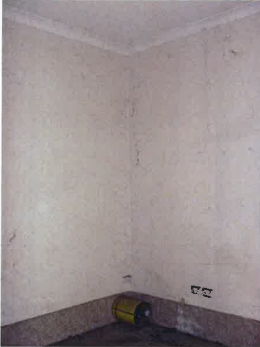
Fig. 26 North section of building.
