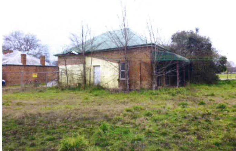
Fig. 34 East and north facades. The demolition of a rear service wing is evident.
