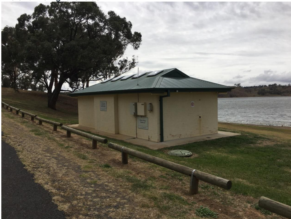
Photo 1: Existing toilet block
