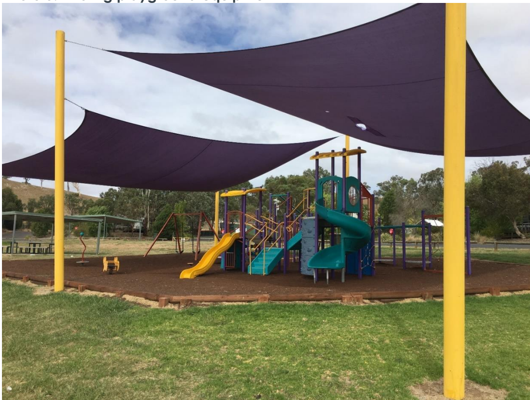
Photo 5: Existing playground equipment
