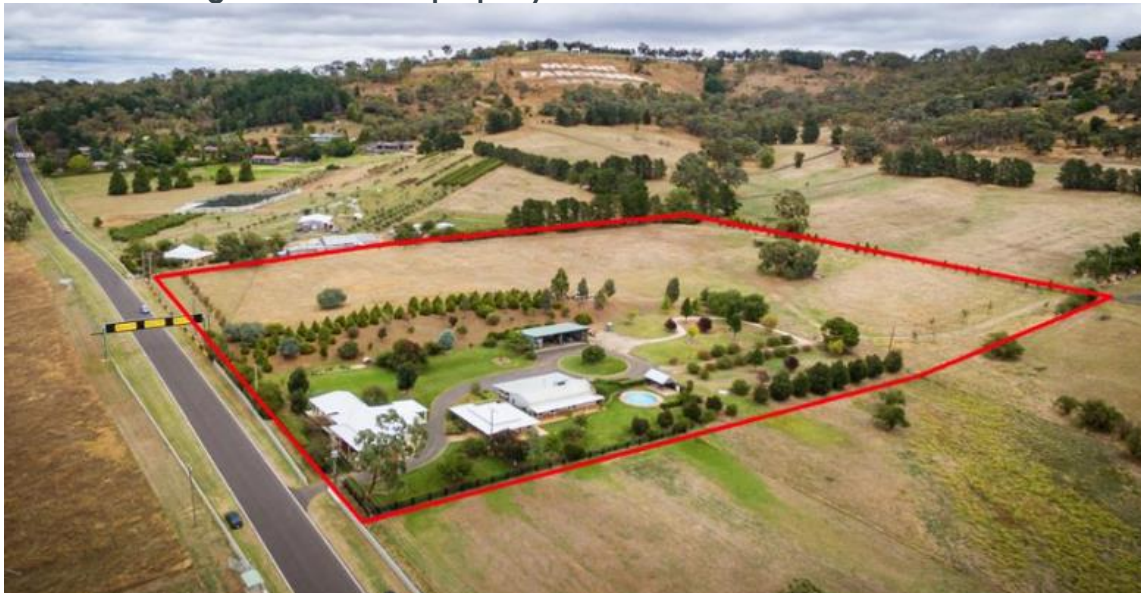
Photo 1: Looking south over the property
