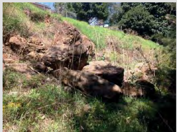
D) Terrace margin with rock protection.
