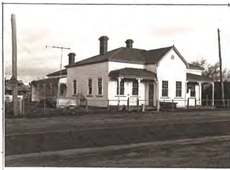
Image: Old house in Wattle Flat, Sofala Road
