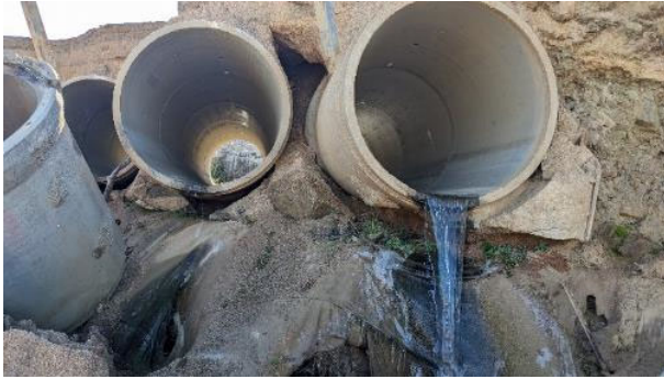
Plate 13 Existing culvert provides potential habitat to mud nesting bird species.
