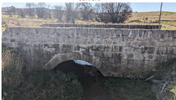
Plate 19 Heritage listed Kellosiel Creek Stone Bridge
