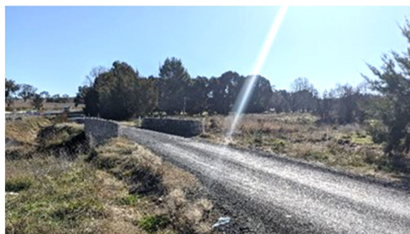
Plate 20 Temporary Freemantle Road diversion across the Kellosiel Creek Stone Bridge
