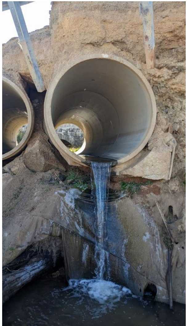
Plate 4 Clear waterflows from Kellosiel Creek culvert were noted during surveys
