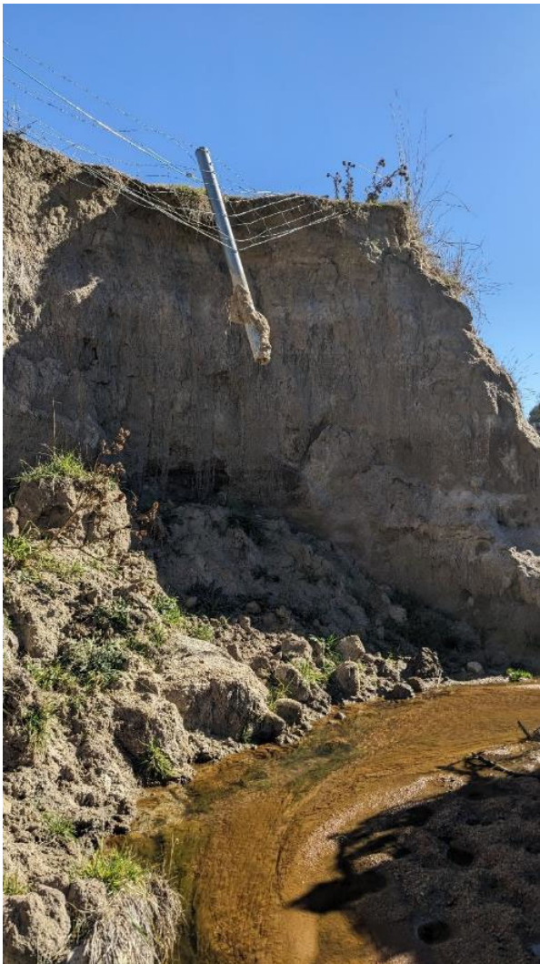
Plate 3 Eroded creek bank along the southern bank of Kellosiel creek
