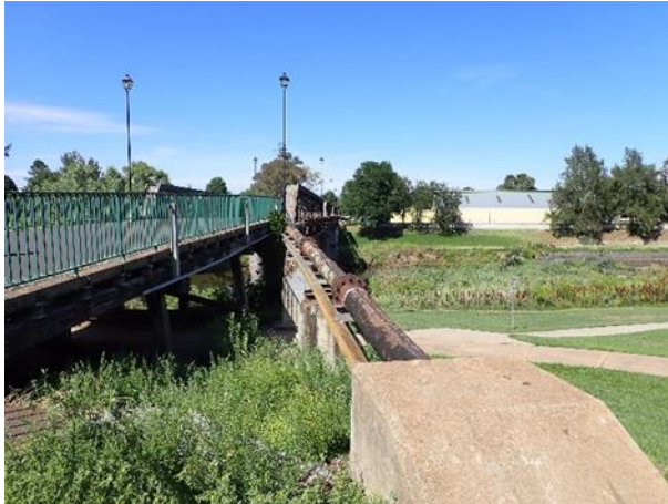
Figure 21 – Service Pipes View From Bridge Deck
