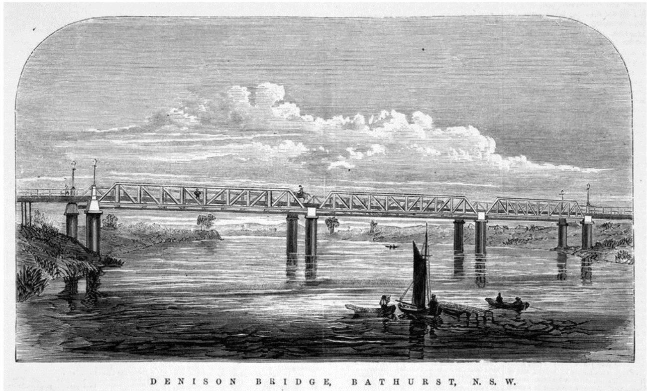
Figure 3 – Denison Bridge Bathurst, NSW c.1872 (source: Trove)
