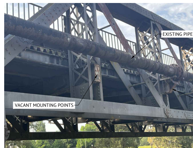
PLATE 1: DENISON BRIDGE PROPOSED PIPE MOUNTING LOCATION
