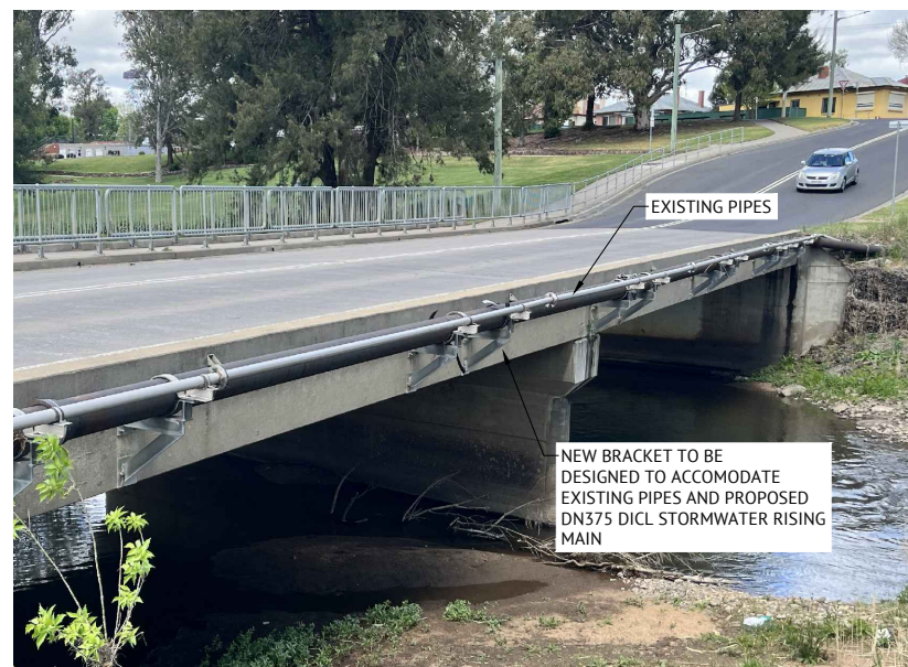
PLATE 2: HEREFORD BRIDGE PROPOSED PIPE MOUNTING LOCATION
