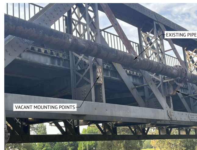
PLATE 1: DENISON BRIDGE PROPOSED PIPE MOUNTING LOCATION
