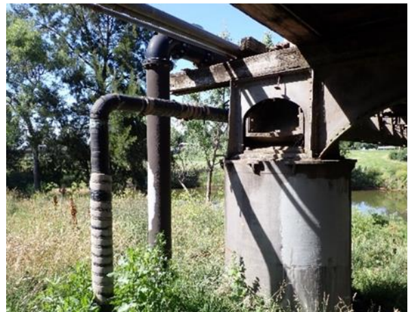
Figure 12 – West Side Service Pipes (Upstream)
