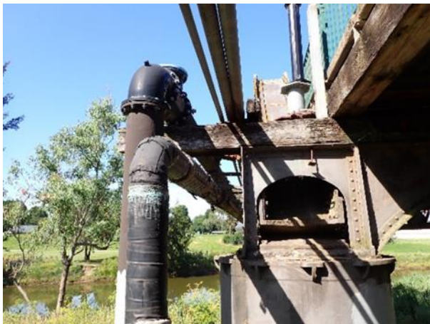
Figure 11 – West Side Service Pipes (Upstream)
