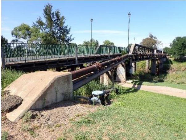
Figure 15 – East Service Pipes (Upstream)
