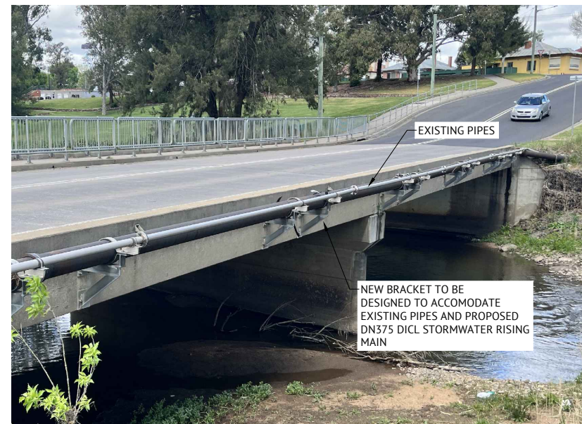
PLATE 2: HEREFORD BRIDGE PROPOSED PIPE MOUNTING LOCATION
